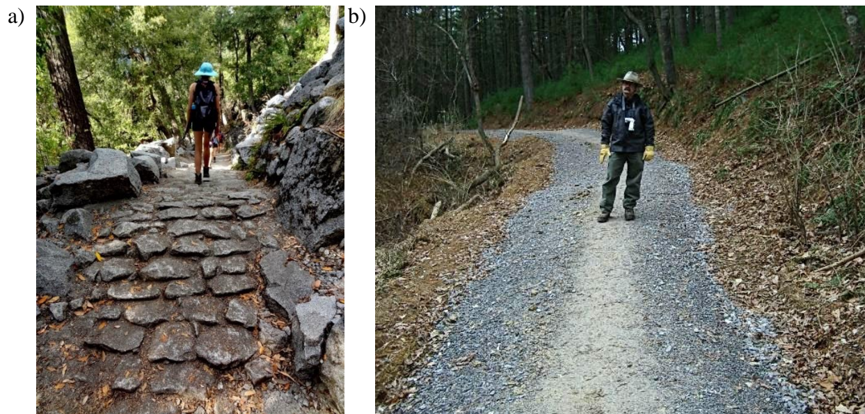
Figure 4. a) Trails that must support heavy traffic, particularly by horses, can be armored with embedded rock. b) Crushed rock (gravel) also supports heavy traffic, though is more easily displaced when wet.
