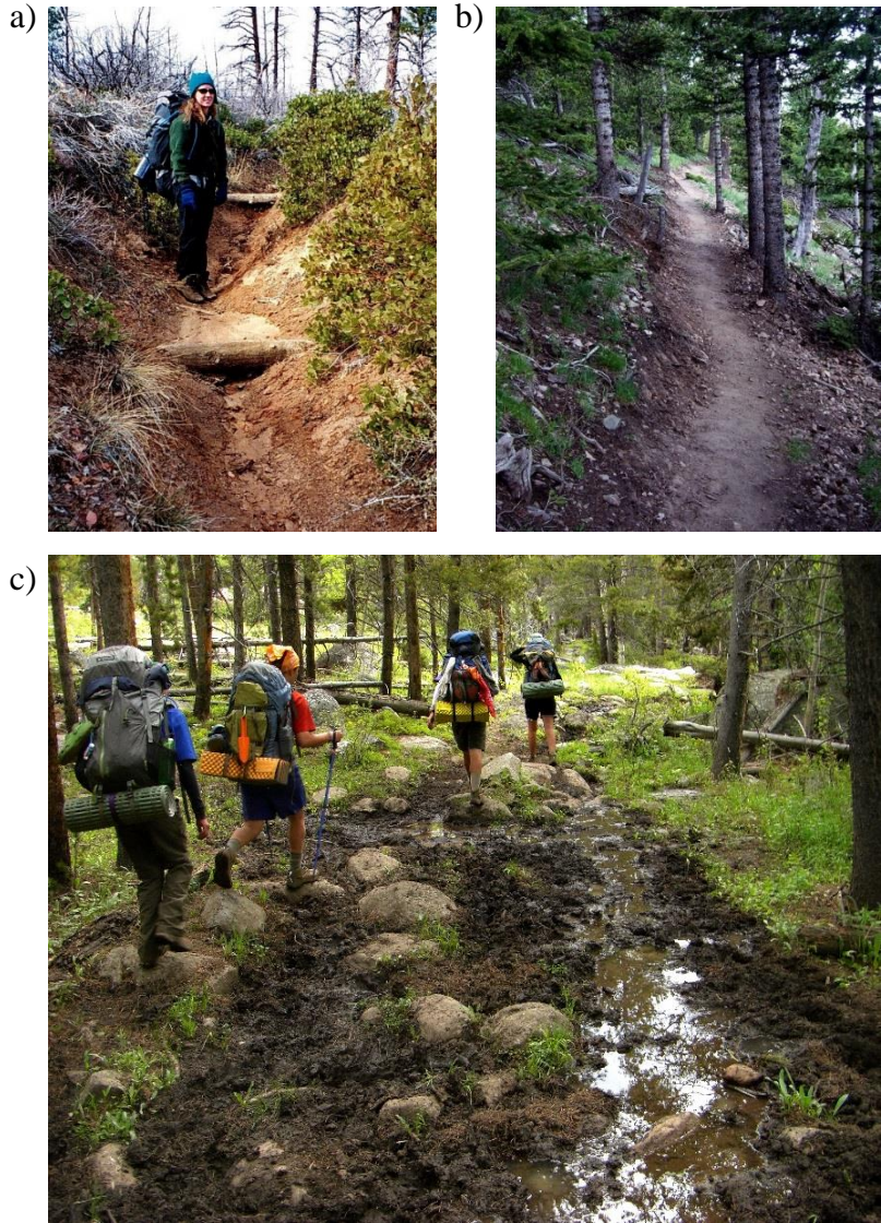
Figure 2. a) Steep fall-line trails (TSA <22^{\circ} ) erode rapidly b) Side-hill contour-aligned trails (TSA >69^{\circ} ) resist widening, muddiness, and soil loss. c) TSA is less influential in flat terrain where trail widening and muddiness are common problems.
