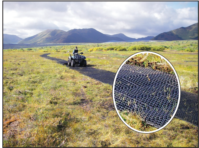
Figure 11–7—A trail-hardened surface of porous pavement panels provides passage over permafrost-associated wetlands on the Karluk River Portage Trail within Alaska’s Kodiak Island National Wildlife Refuge.
