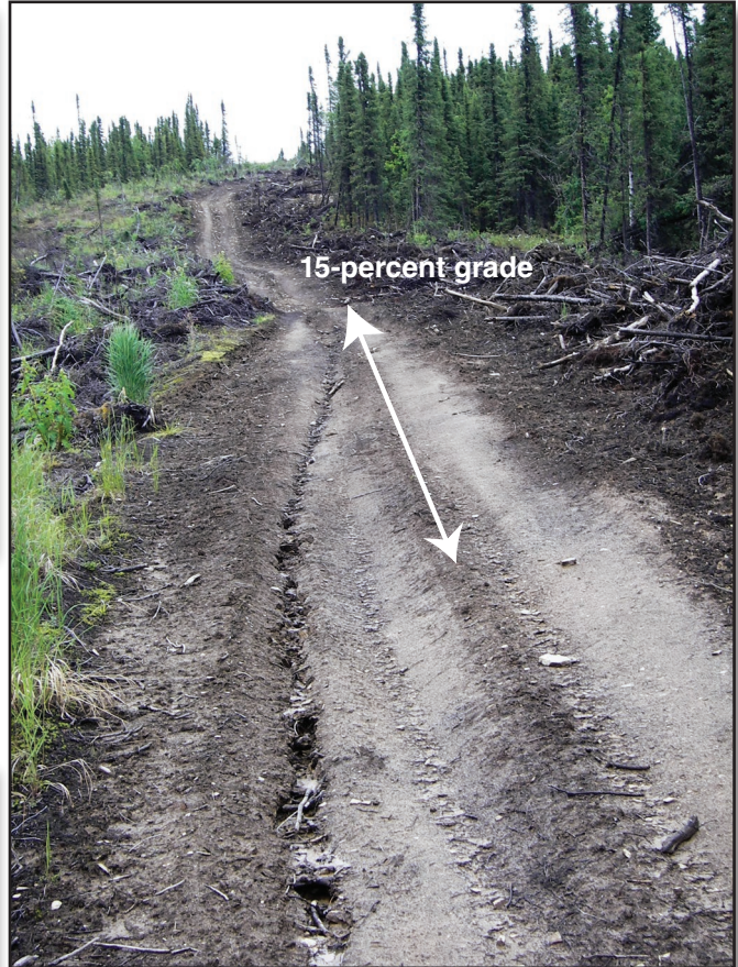
A portion of the ridgetop fireline used to access the Compeau trail. Note the fall-line alignment and lack of integrated water control—a few of the features that limit the sustainability of this adapted trail segment.
