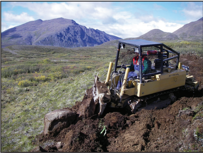
Weighing nearly 10,000 pounds with 83 horsepower, the Sweco 480 (now known as the Sutter 480) is well equipped to handle the many large rocks encountered along the alignment.
