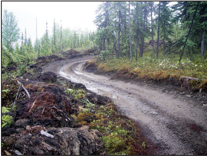
One of several climbing turns. Note the maintained uniform grade through the turn and good vertical separation between the upper and lower approaches.
