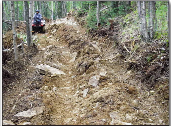
This photo shows an example of the roughed in double-wide, two-tiered pass the Sweco 480 had to make to meet the 8-foot tread width specification.
