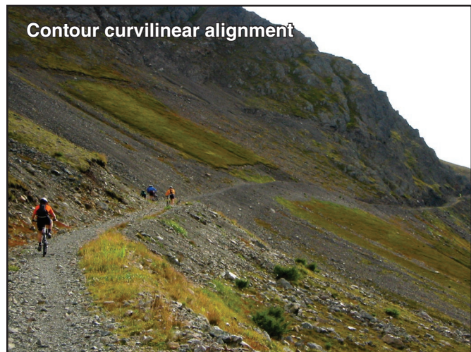
Figure 2–1—This trail in the Chugach National Forest illustrates contour curvilinear alignment, the first sustainable trail design guideline. Note how the trail crosses the slope along the topographic contour rather than running more directly up or down the slope. The sideslope location of the trail and its alignment encourage the natural force of gravity to carry water across the trail rather than directing it down the trail.
