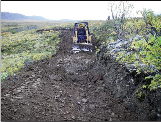
The Glacier Lake Trail was designed as a 7- to 8-foot wide tread with a full bench. The Sweco 480 is digging the grade down to native material to meet the full bench specification.
