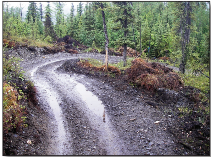
Figure 13–1—Off-highway vehicle (OHV) traffic on this cut-through climbing turn quickly forms wheel ruts and banked turns that can disrupt tread surface drainage. Regrading these to their original specifications is one of the primary purposes of OHV tread maintenance.
