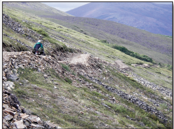
Figure 12–10—This trail displays the stair-step alignment that is characteristic of integrating grade reversals when ascending or descending a sideslope.
