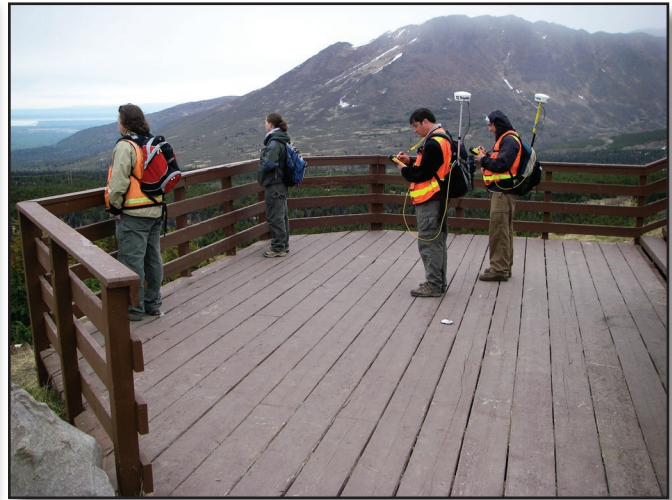
Figure 10-4—Global Positioning System mapping of a deck at a scenic overlook. The deck could be mapped as a point feature to simply denote its location, or as an area feature to document its footprint. Two surveyors are collecting data. The second instrument provides a backup dataset.
