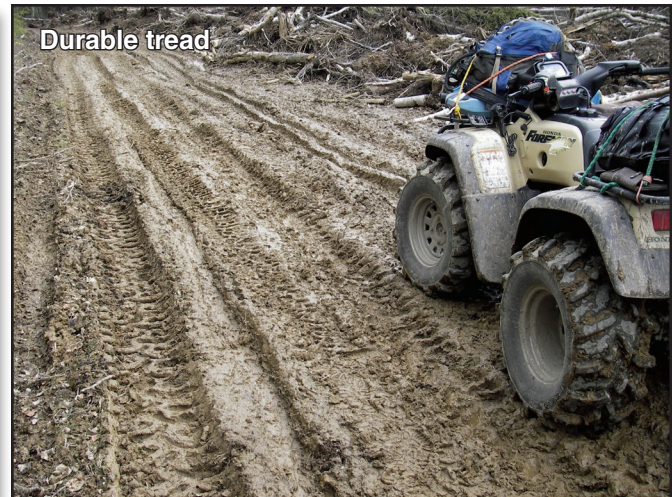
Figure 2-5—This figure illustrates the need for durable tread, the fifth sustainable trail design guideline. Even if contour curvilinear alignment, integrated drainage, and full bench construction are provided, some soils and environmental conditions require that surface tread receive extra attention. This photo of a sustainable off-highway vehicle trail alignment in Alaska's Chena River State Recreation Area illustrates a tread surface that is excessively muddy when wet. Capping this area with gravel would ensure a durable wear surface under all climatic conditions.
