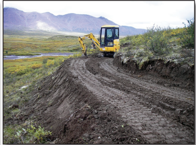
A miniexcavator was used to compact fill slopes, shape backslopes, reduce root wads and place mats of stripped vegetation on exposed soil.
