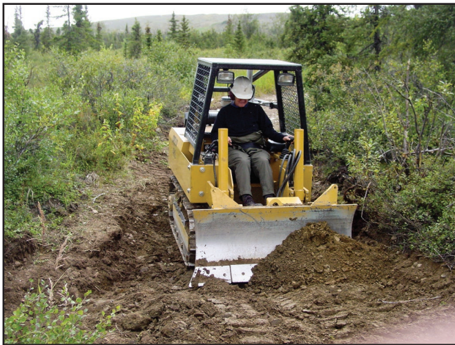
Figure 14–1—A trail dozer is an efficient piece of earth-moving equipment for trail construction and maintenance.
