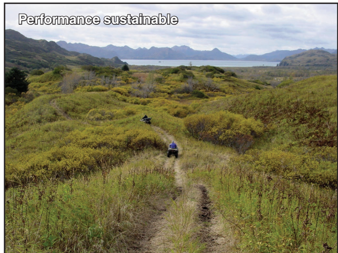
Figure 3–2—An example of a performance sustainable section of the Summit-Lake Miam Trail on Kodiak Island, AK. This section follows a ridgeline that has multiple segments of fall-line alignments. Because of low use levels there is little degradation, but continued or increased use could lead to erosion and rapid degradation.
