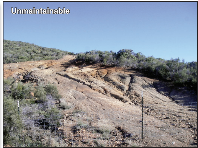
Figure 3-4—An example of an unmaintainable trail section. This section has none of the sustainable trail design elements and displays evidence of extreme degradation. The section has been closed and slated for reclamation.
