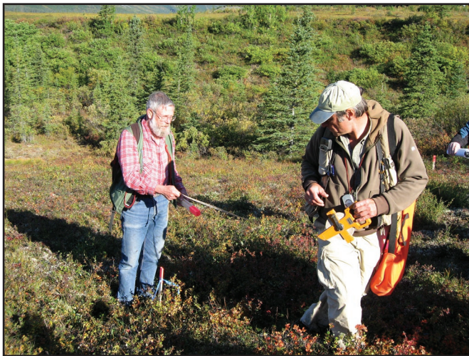
Figure 12–9—Measuring the turn radius with a tape is the best way to ensure that the sideslope area is large enough to accommodate the entire climbing turn layout.
