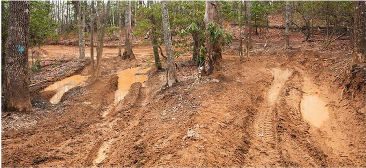
Damage to forest roads similar to Water Tower and Moss Falls Trails
